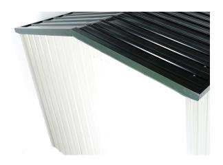
Step 2: Centralise Barge Flashing on gable end and rivet in place, one rivet into every second Rib. Fit two rivets through top of Barge into Rib. Repeat with other Barge Flashing. Check Spoutings are straight, then rivet to Roof one rivet every second Rib.
