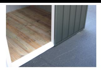
Step 4: Nail in each Floor Board, two 50mm nails in each end and two into Joists. Measure and cut Floor Flashing (110) to fit in between Door Jamb Flashings and nail in place using 50mm Clouts.
