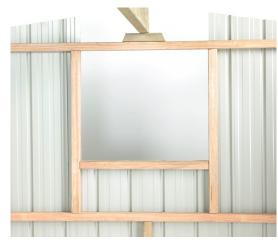
Step 2: On the inside of the shed, position studs and Nog centrally on window opening. Make sure the studs are parallel and nail into Top Plate and End Wall Nog.
