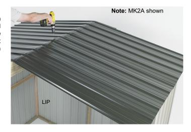
Step 3: Starting from the left hand end, centralize Roof on Ridge Beam. Ensure Roof is tight against end Wall Sheets, predrill then nail one 50mm Clout through Rib into the Ridge Beam. At the back, line up Ribs on the Roof Sheet with the Ribs on Wall Sheet. Using one 50mm Clout, nail through Rib into Back Top Plate. Repeat at the front.
