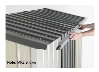
**Step 1:** Position Barge Flashing (A102) on gable ends. Position a Spouting (A103) and rivet to the Barge Flashing at each end. Repeat with other Spouting.
