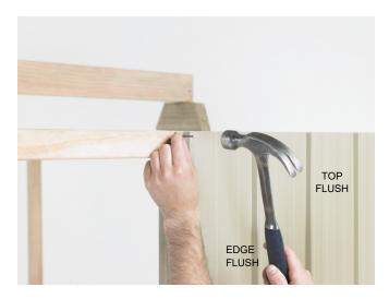
Step 2: Back Wall: Position the first Wall Sheet with the LIP on the right hand side. Ensuring the LIP is flush with the side of the corner Stud and the top of the Wall Sheet is flush with the top of the Top Plate, tack in place. Position the next Wall Sheet with the LIP on the right hand side. Overlap as shown in *fig 1*. Ensuring Wall Sheet is flush with top of Top Plate, tack in place.
